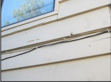
Natural wood siding has some knot holes. Consider caulking or, at the very least, monitoring for the presence of insects, bird damage, or other activity.
