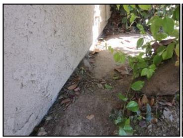
Maintenance Tip: When landscaping, keep plants, even at full growth, at least a foot (preferably 18 inches) from house siding and windows. Keep trees away from foundation and roof. Plants in contact or proximity to home can provide pathways for wood destroying insects, as well as abrade and damage siding, screens and roofs.
