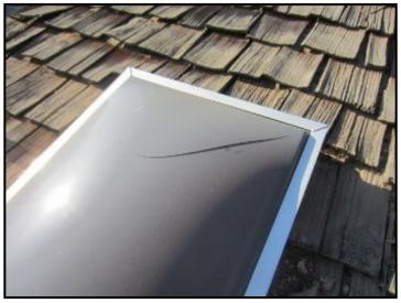
The sky light is past its serviceable life time and shows signs of excessive leaking, have it replaced/repaired by a qualified individual.
