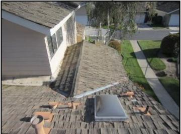
Maintenance Tip: Roof design has many peaks and valleys; keep roof cleared of debris to extend life of roof.
