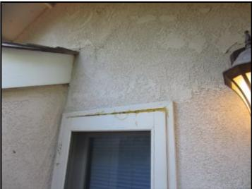
Bathroom exterior door with expanded foam seal
