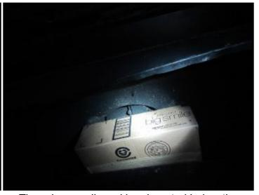
There is a cardboard box inserted below the damper apparently in an attempt to keep the damper closed. Strongly recommend that a qualified chimney sweep evaluate/repair before this unit is used.
