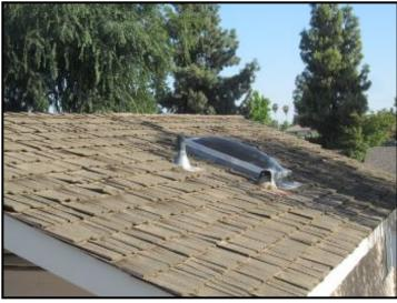
Some wood shakes missing / damaged / nails lifting.
