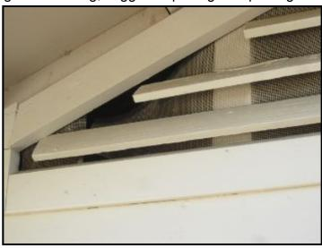
Vent screens are damaged or missing, suggest repairing or replacing screens as necessary.
