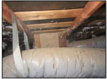
Missing insulation at skylight shafts
