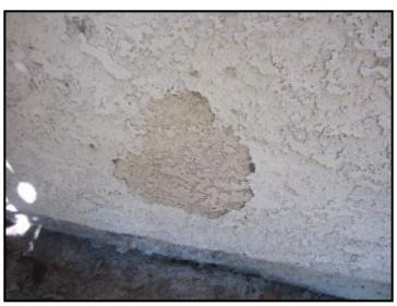
There are a few holes and cracks in the stucco. There is a small area on the west wall that the paint finish is peeling. Recommend monitoring and repairing as necessary
