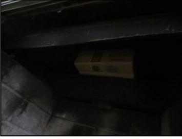
There is a cardboard box inserted below the damper apparently in an attempt to keep the damper closed. Strongly recommend that a qualified chimney sweep evaluate/repair before this unit is used.
