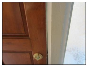
Weatherstripping is not sealing at most exterior doors
