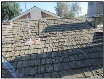
Wood shake roof is beyond functional lifespan. Recommend replacing the roof.
