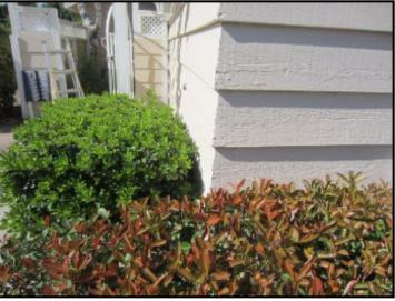
Maintenance Tip: When landscaping, keep plants, even at full growth, at least a foot (preferably 18 inches) from house siding and windows. Keep trees away from foundation and roof. Plants in contact or proximity to home can provide pathways for wood destroying insects, as well as abrade and damage siding, screens and roofs.
