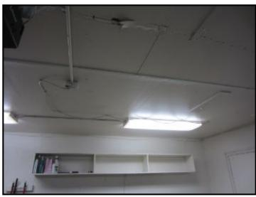
Surface mounted flourescent lights have been wired with cord & plug. Recommend hard wiring per acceptable standards.
