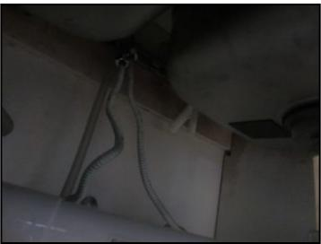
Lack of a proper air gap noted at dishwasher drain line. In the event of a sewer backup this device prevents sewer matter from entering into dishwasher. Recommend having a qualified plumber install a air gap to prevent possible contamination.
