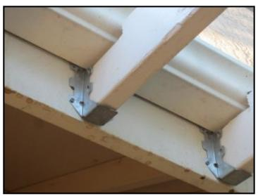
The rafters of the lattice patio cover are attached to the house fascia with screws from the back side. There has been an attempt to fit the rafters with joist hangers, but the proper fasteners have not been used. Recommend having a qualified contractor complete the installation of joist hangers using the proper fasteners.
