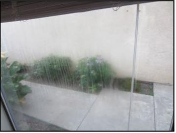
One or more window/s shows sign of loss of seal/condensation, recommend repair or replace to provide energy savings and prevent hazed window from limiting view out of window.
