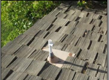
Condensate lines are missing from both roof-top dual pack units, draining condensate onto roofing. This will reduce the life of the roofing and create potential roof leaks. Recommend having a qualified HVAC contractor evaluate and repair.
