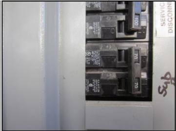
Main Electrical Panel cover does not appear to be the original cover and does not fit well inside panel. Gaps are present at side of breakers. Recommend having a qualified electrician evaluate and repair.
