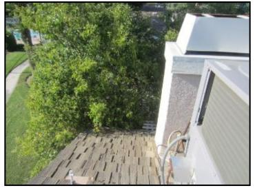
Tree limbs within 10 feet of roof should be trimmed away to provide air and sunlight to roof, while minimizing debris & dampness.
