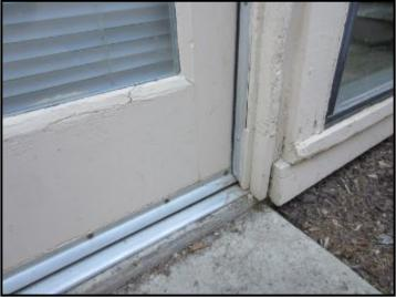
Wood deterioration observed at east door out of living room. Suggest repairs/replacement as needed.
