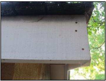
Fascia at northeast corner of house has been replaced recently, but non-galvanized nails were used to attach it. These nails will rust and stain the paint finish. Recommend removing the GV sinker nails, and re-nail fascia with hot-dipped galvanized nails or screws.
