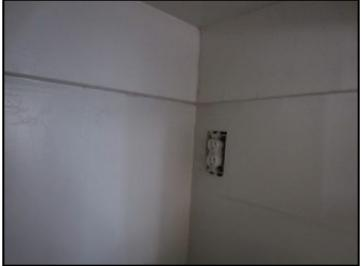
Outlet cover plates missing. Under stairs
