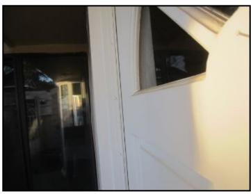
Doors do not seal well. this can be an energy drain.
