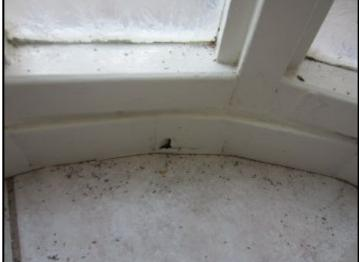
Deterioration of wooden frames noted. While basic maintenance may prolong the life of these window frames, replacement may be necessary at some point.
