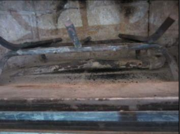
Gas log lighter is damaged and should be repaired/replaced prior to using.
