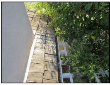
Clean gutters: Significant amounts of debris evident.
