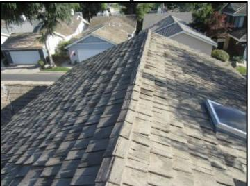
Some wood shakes missing / damaged / nails lifting.
