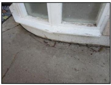
Front sidewalk settling away from house under entry door windows. Monitor for additional movement.
