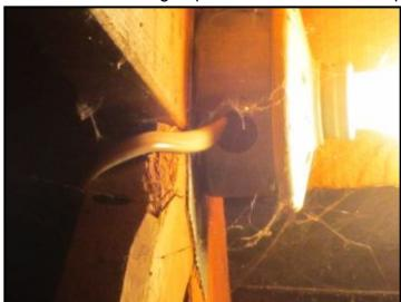
Attic switch and light boxes both have romex wiring with no connectors to metal boxes. Recommend having a qualified electrician make proper connections.
