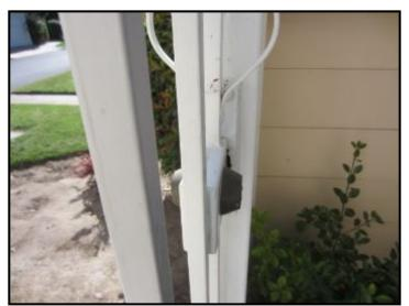
Double cylinder lock on front gate does not provide adequate emergency egress
