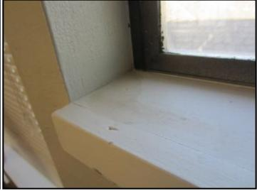
Evidence of past leaking on window sills @ stairway windows
