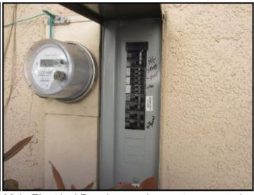
Area 3' in front of electrical panels should be kept Main Electrical Panel cover does not appear to be clear for access the original cover and does not fit well inside panel. Gaps are present at side of breakers. Recommend having a qualified electrician evaluate and repair.
